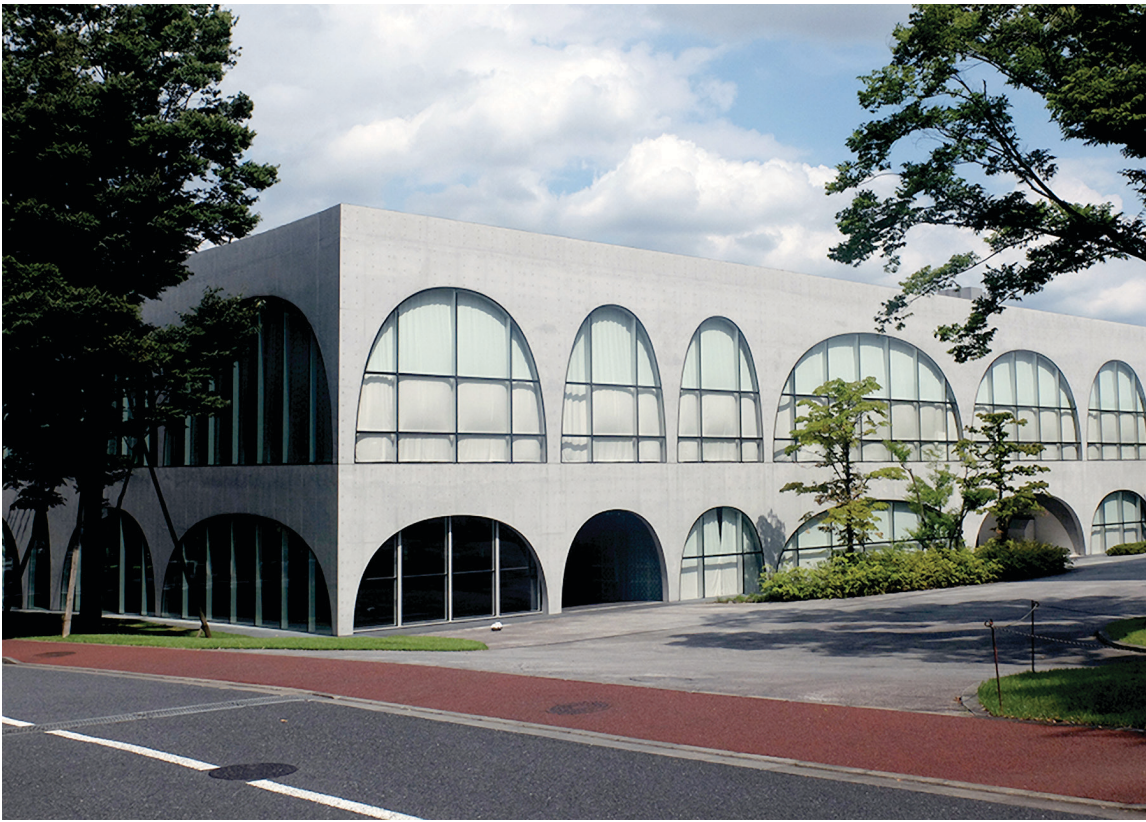
Figure 1. The library of Tama Art University's campus in Hachioji, Tokyo, was designed by renowned Japanese architect Toyo Ito.
